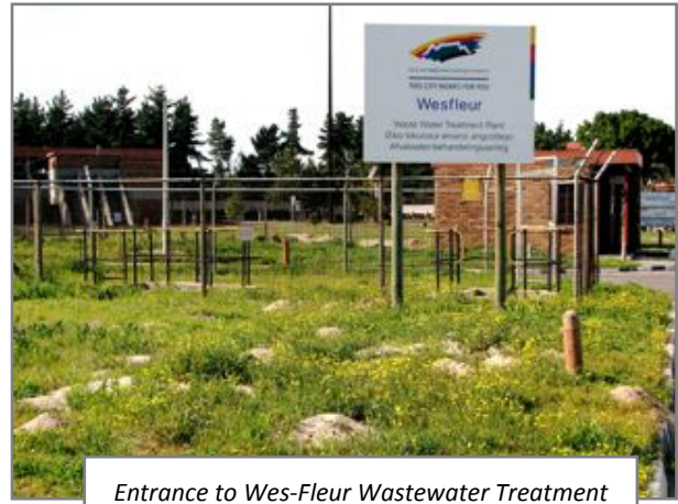
Entrance to Wes-Fleur Wastewater Treatment Works with domestic WWTW in background.
