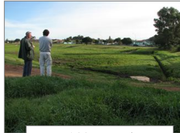
Basin 3: Storm water outlet.
