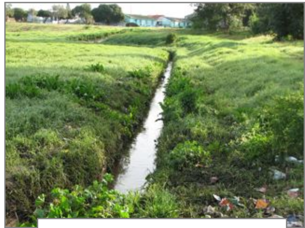
Basin 3: Low level flow channel.
