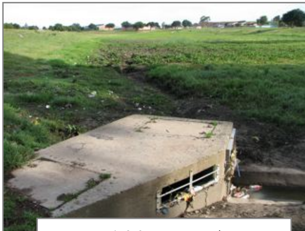
Basin 3: Storm water outlet.
