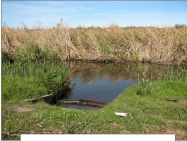
Basin 9: Industrial storm water detention.
